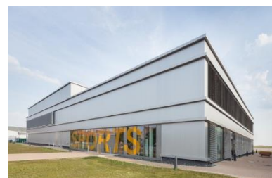
Physical Fitness Center, Katterbach
